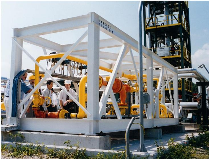
Results taken from the system instrumentation confirmed an impressive boost to the low pressure produced fluids. At the discharge of the system, measurements showed that the low pressure fluids had been boosted to a new range of pressures of 56 barg (744 bbl/d) to 58 barg (6048 bbl/d) representing a gain in pressure of up to 25%.
